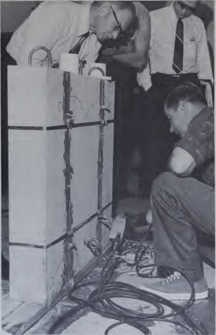
Figure 187.—Demonstration of a proprietary epoxy grout injection system for repairing cracks in concrete structures. P801-D-75011.
